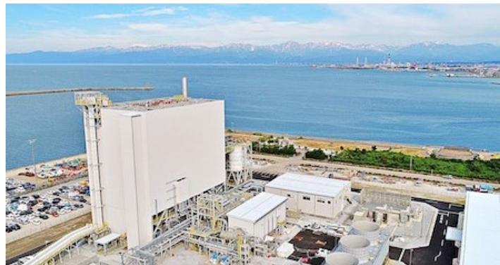
Image-3 Project BE-01 Fushiki Manyofuto Biomass Power Plant
